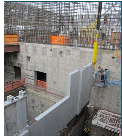
A Pacific Northwest business manufactured several of the Vit Plant's massive shield doors, including a 102-ton door installed in the Pretreatment Facility.
