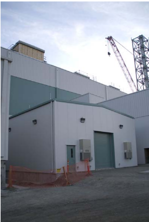
The Low-Activity Waste Vitrification Facility switchgear building (in the foreground) will serve as the facility's primary power source and will house enough electricity to power nearly 1,800 residential homes.
