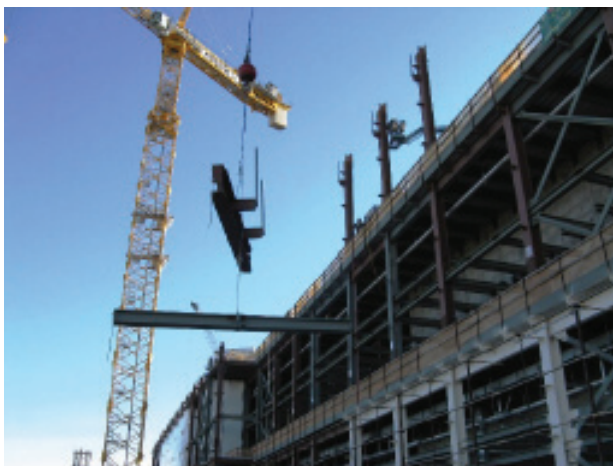
The Pretreatment Facility now reaches 85 feet in places.
