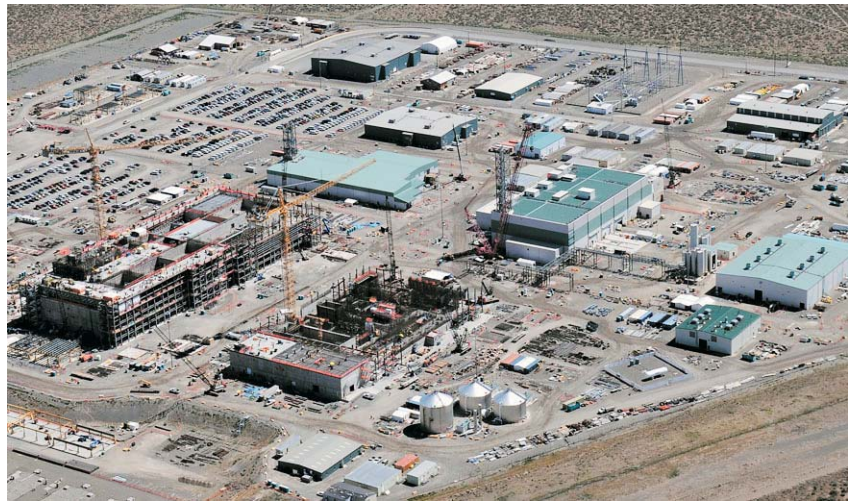
WTP in July 2010
